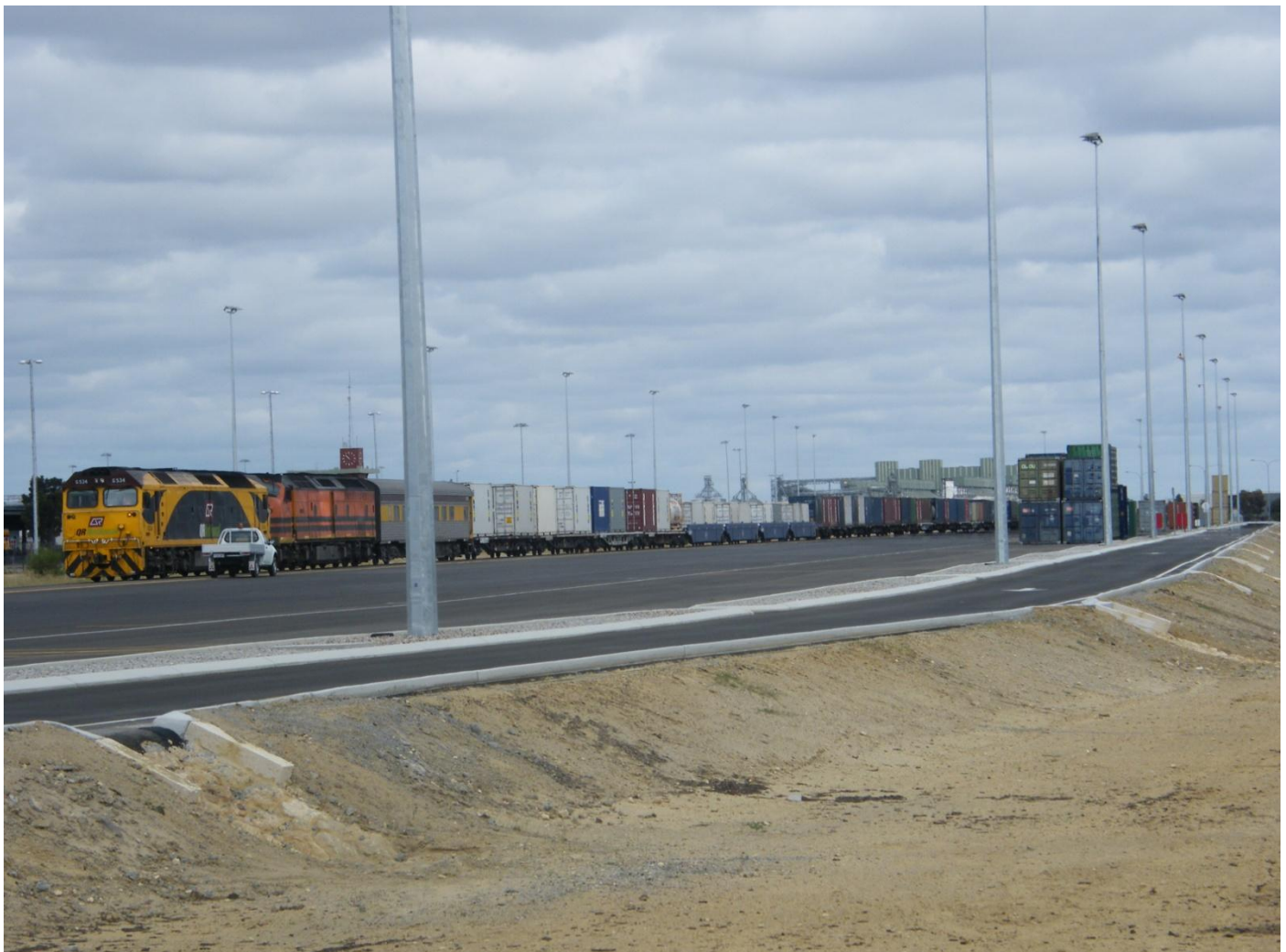
G534 & CLP10 on 7API QR National intermodal service to Adelaide in the new QRN intermodal terminal at Forrestfield this is first train to depart this facility on April 25th following it opening. Photo Jim Bisdee
