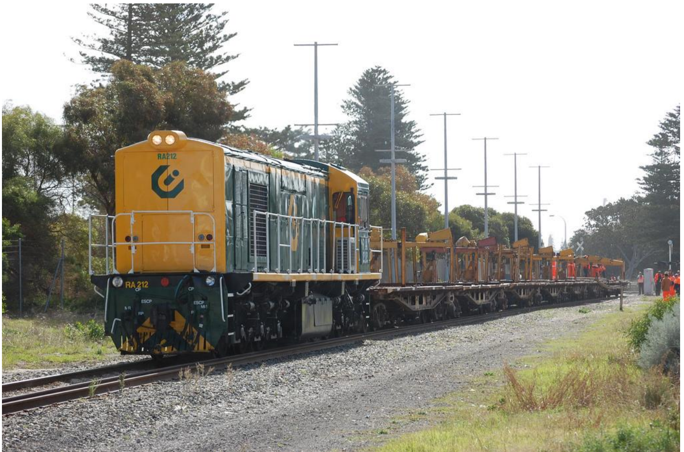
RA212 on vacuum braked rail train dropping rail on the Fremantle to Cockburn Junction line at South Beach station that was built for Americas Cup regatta in 1986/87 and unused since. Photo Brendan Cherry
