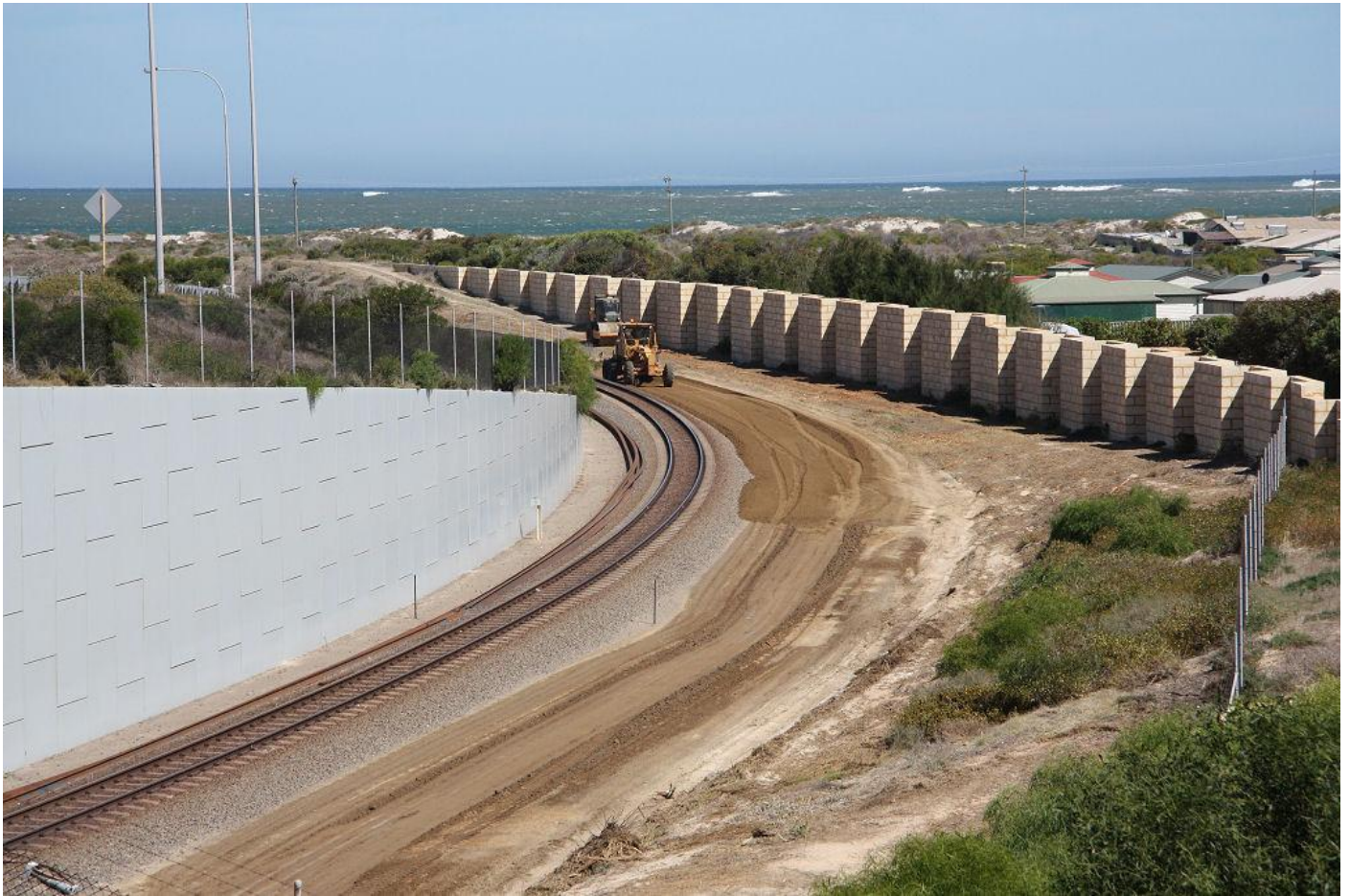
Earthworks March 29th for the second track to be laid through tunnel at Geraldton port. Photo Phil Melling
