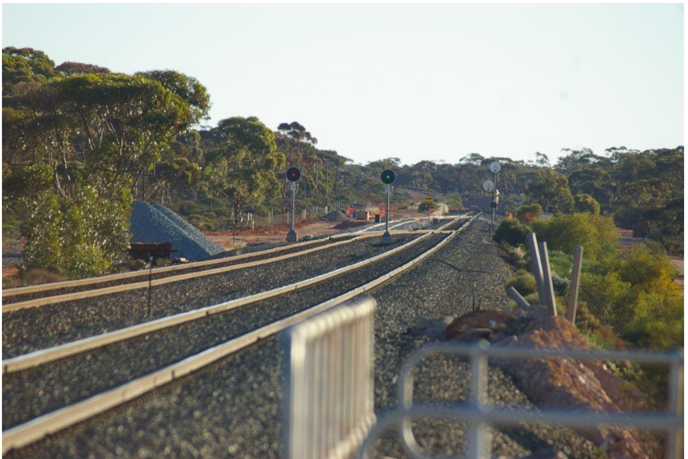
Western end of Binduli triangle April 5th with some 500 metre extension completed as part of trackwork to allow introduction of 159 wagon ore trains from Koolyanobbing to Esperance.
