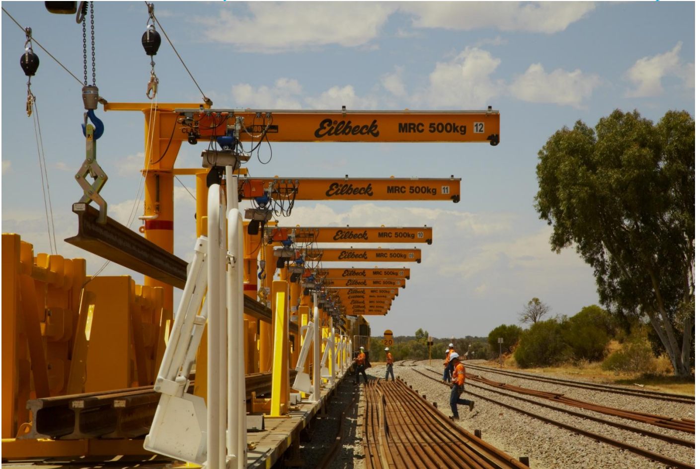
Rail being loaded onto rail train at Mullewa on October 21st.
