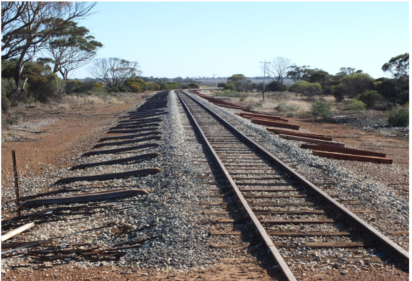
New steel and wooden sleepers laid out ready to be inserted in the track north of Ballidu 12/05. Photo Jim B
