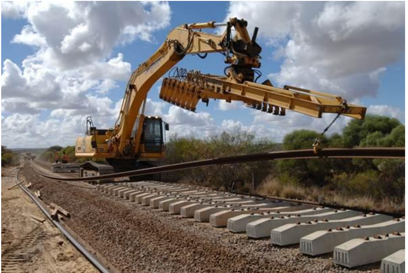
Lifting rail onto the dual gauge sleepers as part of the Narngulu Mullewa upgrading. Photo Brookfield Rail
