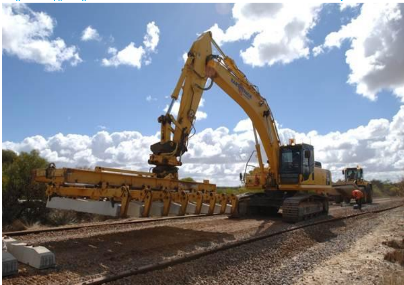
Mechanical sleeper laying onto prepared track bed as part of the track upgrading. Photo Brookfield Rail
