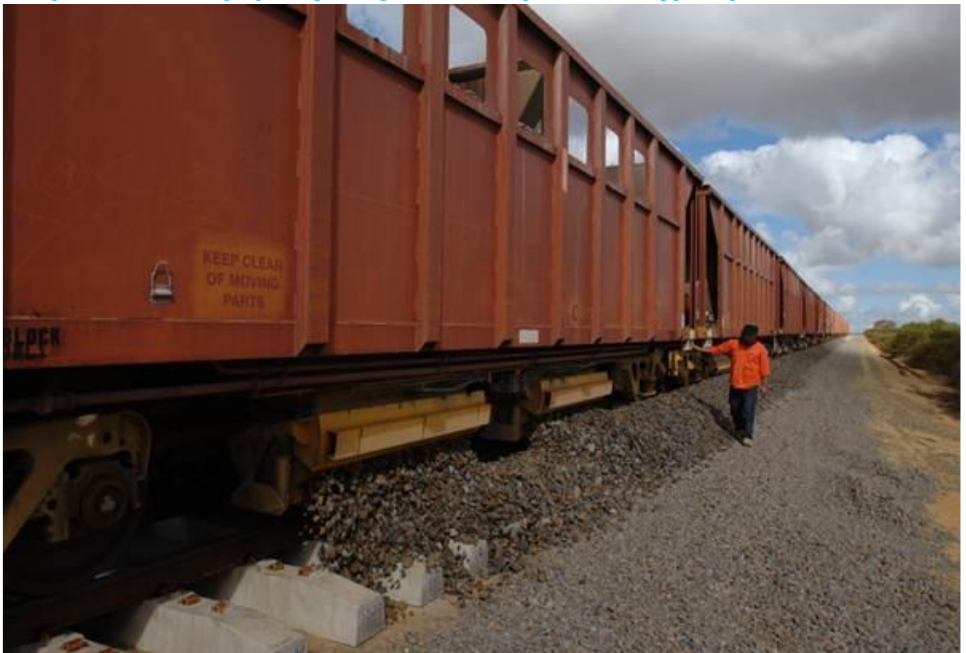
Initial ballasting of freshly upgraded track on Narngulu Mullewa line.
