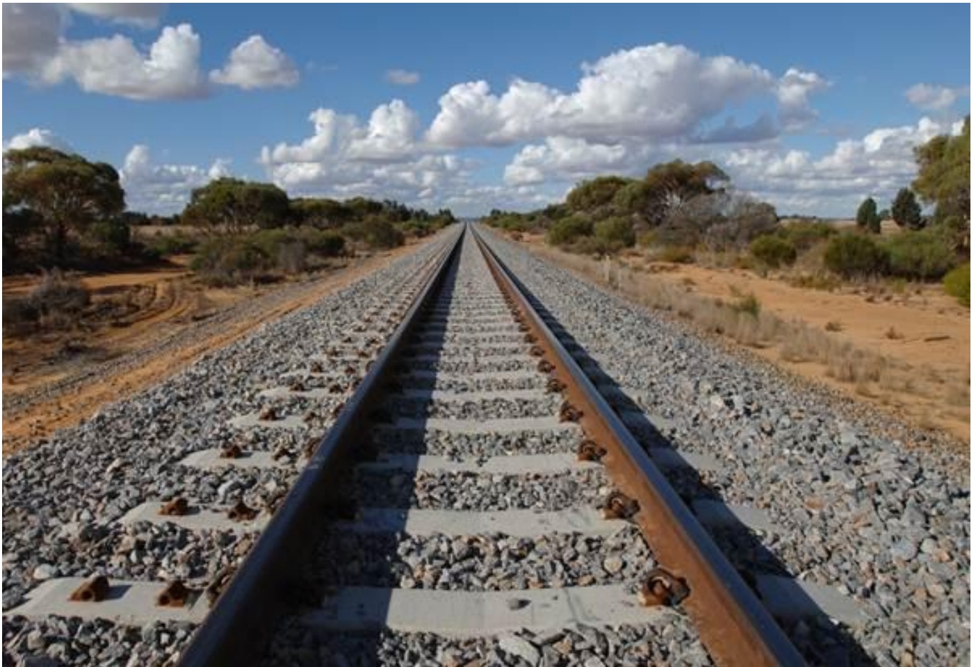
Completed upgraded section of line with close spaced dual gauge concrete sleepers. Photo Brookfield Rail
