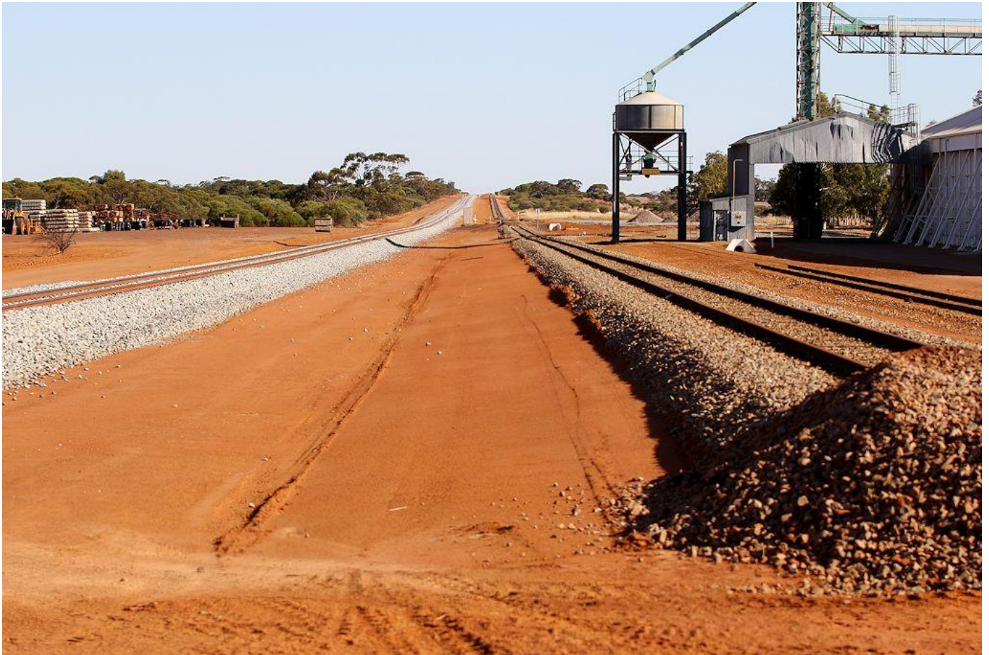
Pintharuka CBH Grain Bin is now no longer connected to rail with new heavy duty line on left and old line on the right still connected to the bin November 17th. Photo Phil Melling
